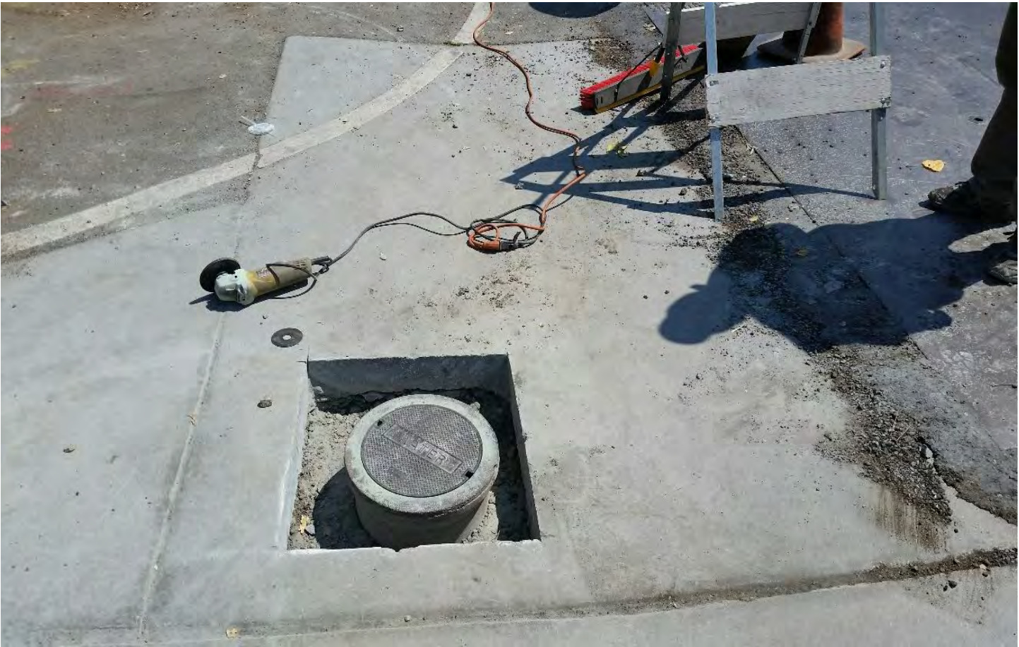
Location: Intersection of Poplar Avenue & East Bayshore Road (August 24, 2016) Picture 2 of 2
