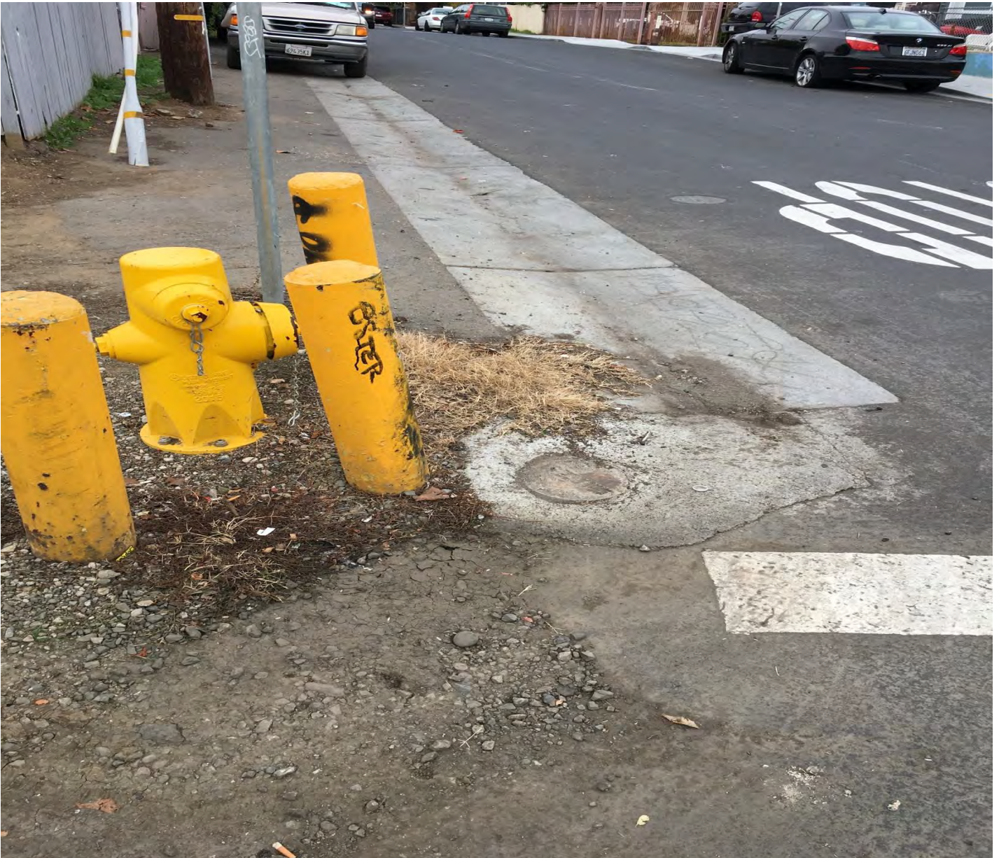
Location: Intersection of Oakwood Avenue & East Bayshore Road (photographed 12/5/16)
