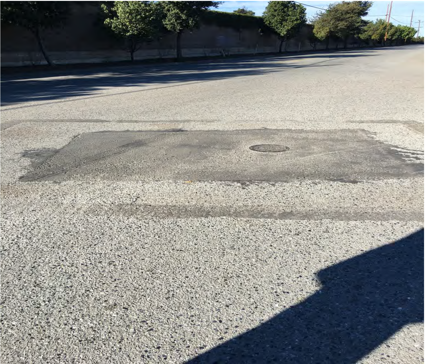
Location: Intersection of Lincoln Street & East Bayshore Road (photographed 12/2/16)
