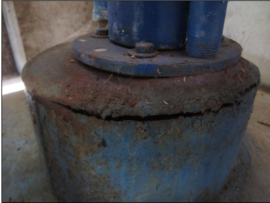
Figure 1. Well 2 – Opening between well casing and top flange.
