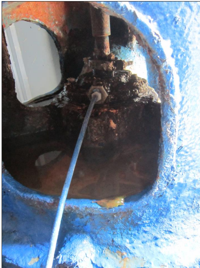
Figure 2. Well 5 – Rust on above ground features.
